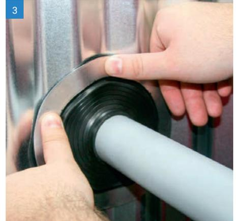
3 Press Master Flash® Low Profile down, bending it to conform to roof profile or irregularities. A blunt tool will help to form flashing to tight roof angles.
