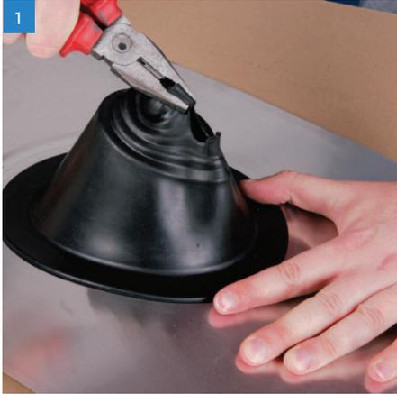
1 Select an appropriate Master Flash® Residential with a pipe range that goes below and beyond fitting. If necessary, follow the lines clearly shown on the flashing and use pliers to pull the tab to create an opening 20 - 30% smaller than pipe diameter. For the steep roof slopes or higher corrugation of the profile, bigger size of Master Flash® should be chosen.
