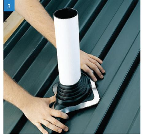
3 Press Master Flash® down, bending it to conform to roof profile or irregularities. A blunt tool will help to form flashing to tight roof angles.
