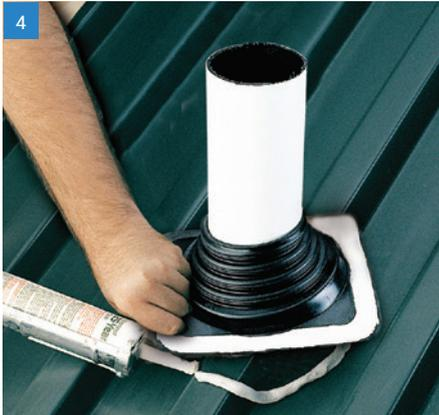
4 Apply sealant between the base of the flashing and the roof.
