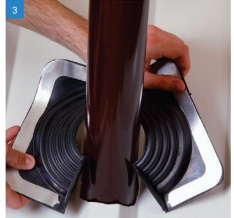
3 Slide the Master Flash® Multi-Flash down the pipe, using a non-petroleum-based lubricant to ease installation. For Retrofit applications, wrap the product around the pipe.
