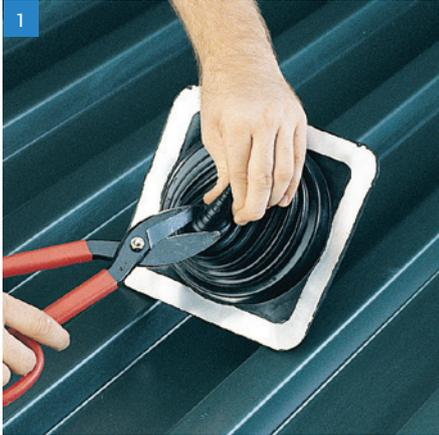
1 Select an appropriate Master Flash® Standard with a pipe range that goes below and beyond fitting. If necessary, use the lines clearly shown on the flashing to trim an opening 20 - 30% smaller than pipe diameter. For the steep roof slopes or higher corrugation of the profile, bigger size of Master Flash® should be chosen.
