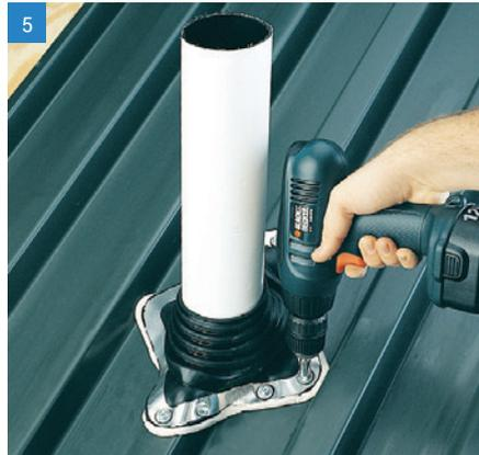
5 Use fasteners to complete sealing. For a secure installation, fastener spacing must not exceed 1.5" (38 mm).
