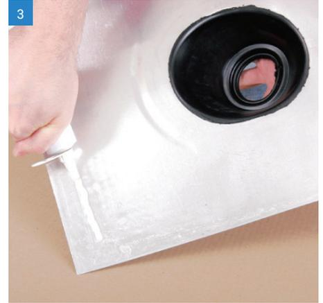
3 Apply sealant on the underneath of the metal base
