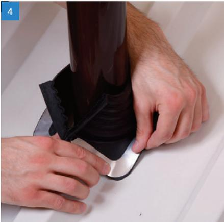
4 Press Master Flash® Multi-Flash down, bending it to conform to roof profile or irregularities. A blunt tool will help to form flashing to tight roof angles.
