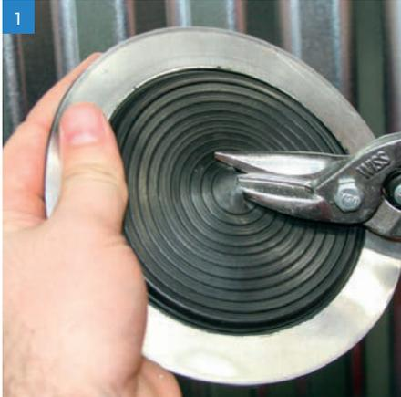
1 Select an appropriate Master Flash® Low Profile with a pipe range that goes below and beyond fitting. If necessary, use the lines clearly shown on the flashing to trim an opening 20-30% smaller than pipe diameter.
