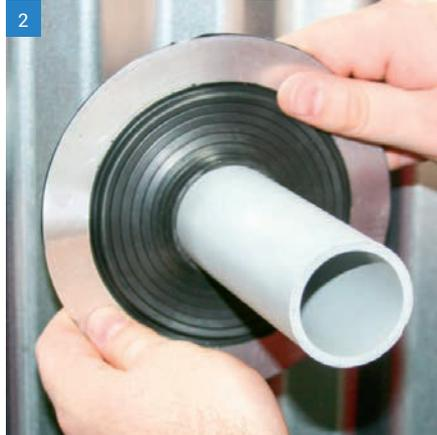
2 Slide the Master Flash® Low Profile down the pipe, using a non-petroleum-based lubricant to ease installation.
