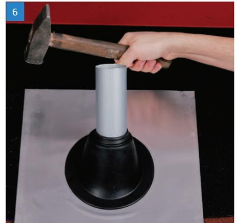
6 Secure and fasten the metal base to the roof.
