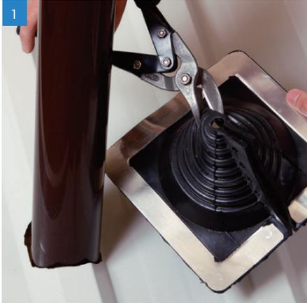
1 Select an appropriate Master Flash® Retrofit with a pipe range that goes below and beyond fitting. If necessary, follow the lines clearly shown on the flashing and create an opening 10-20% smaller than pipe diameter. Slice down the flange. For the steep roof slopes or higher corrugation of the profile, bigger size of Master Flash® should be chosen.
