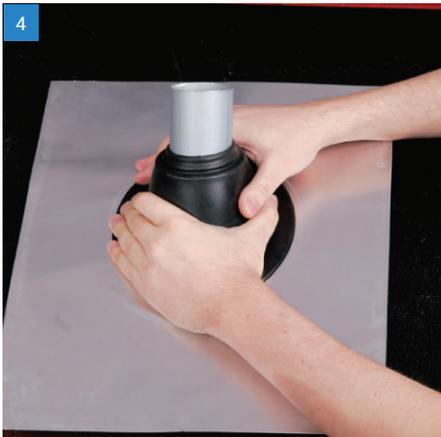
4 Slide the Master Flash® Residential down the pipe, using a non-petroleum-based lubricant to ease installation.
