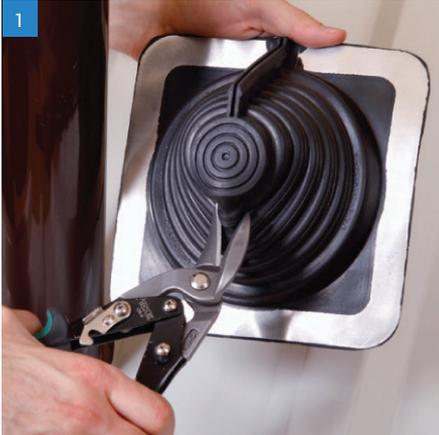
1 Select an appropriate Master Flash® Multi-Flash with a pipe range that goes below and beyond fitting. If necessary, follow the lines clearly shown on the flashing and create an opening 20-30% smaller than pipe diameter. For the steep roof slopes or higher corrugation of the profile, bigger size of Master Flash® should be chosen.
