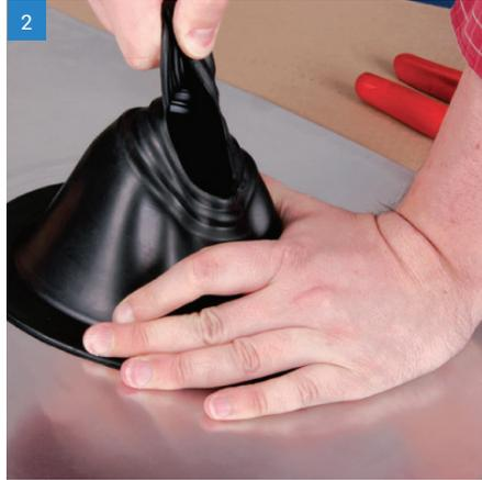
2 Finish adjustments to flashing opening by hand.
